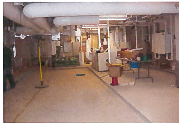
HAWLEY BOILER / HVAC PHASE I PROJECT
